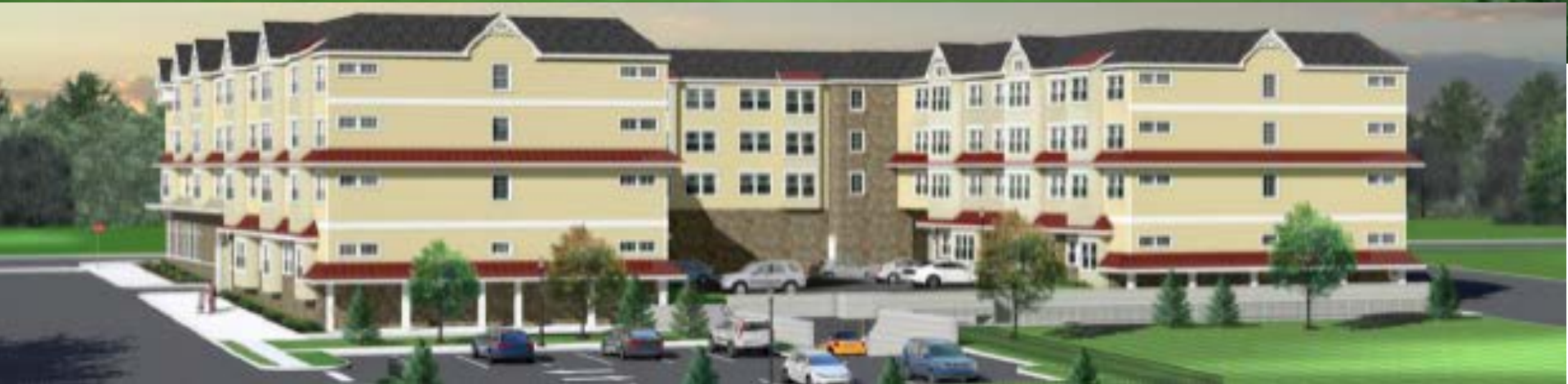
New Jersey UBF new Center & Accommodation
